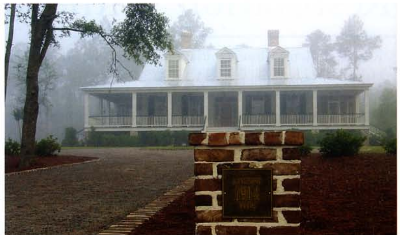
The completed Langford House is seen here from the front drive. The new addition of the partially enclosed wraparound porch takes its cue from what was a traditional practice in the 1920s. In sum, the old house and the new porch together make good on the driving philosophy behind the project: What was old is new again, and vice-versa. Materials were carefully chosen to reflect the period of the original farmhouse and include the seamed-metal roof and custom-milled windows and doors by Fracasso Custom Woodworking, Walterboro, S.C.
